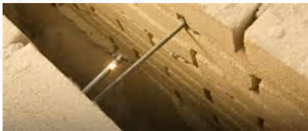
Fig. 13: spouwankers
